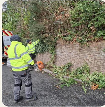
Vegetation clearance along a boundary wall
