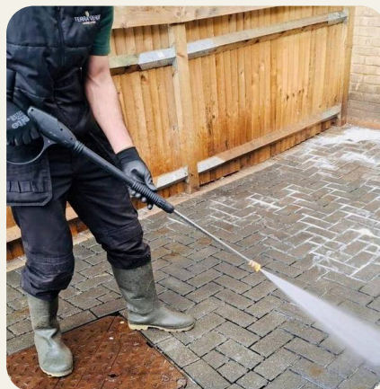
Power washing paved areas
